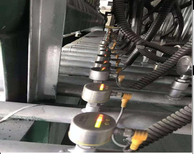
Because the previous brand often failed in the beginning, and also the price is increased. All flow sensors are installed on the cooling water pipes to monitor whether the cooling water stop flowing.
